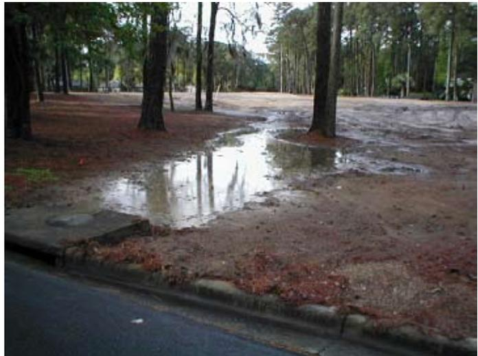
Stormwater runoff from construction area to sewer catch basin in southeastern Georgia.
