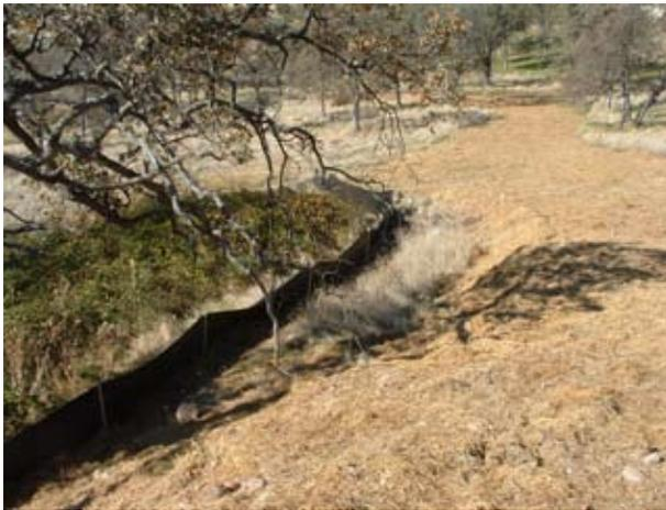
Silt fences and straw mulch distributed over disturbed soils reduce erosion.
